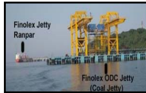
(Photo Courtesy: Finolex) Finolex Main Jetty and Coal Jetty
