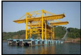
Finolex Coal Jetty and Conveyor Belt
