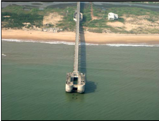
Nagarjuna Sea Water Intake Pier
