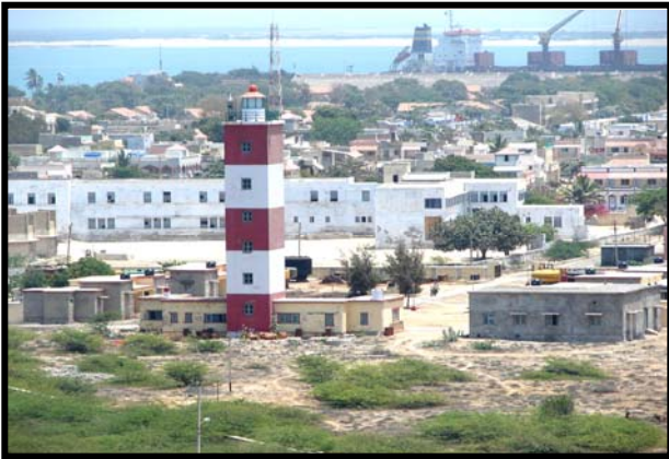
Okha Light House (F 0388)
